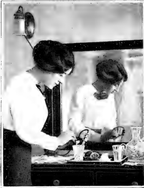
A glass of water may be heated almost instantly by immersing the cylinder in the water
